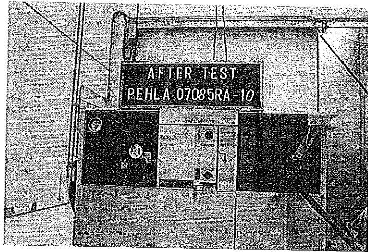
Photo No. 07 After test PEHLA 07085Ra / 10
